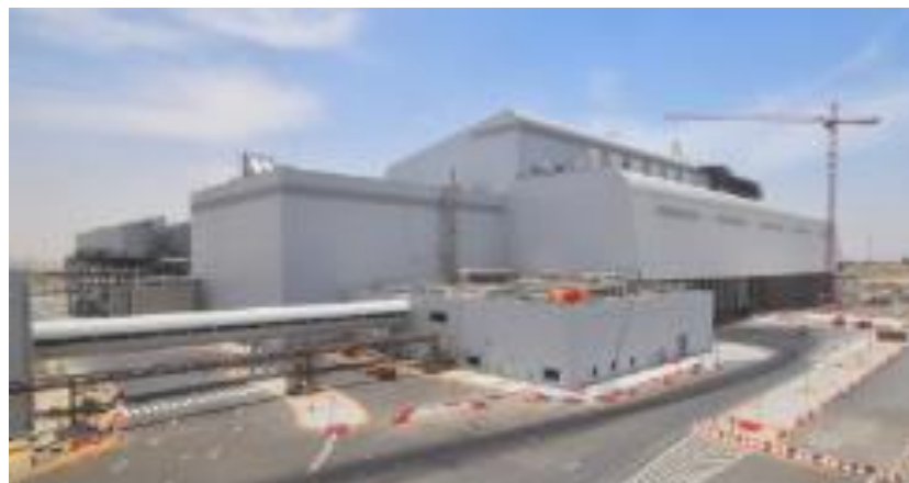
Dubai/UAE, world's largest WtX plant, (1'890 kt/a, 193 MW el ), BOO, in operation
