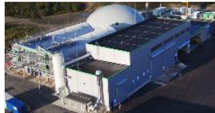
Jönköping/SE, Kompogas® dry AD plant, (40 kt/a, 35 GWh/a CBG), BOO, in operation
