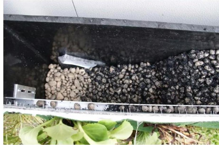
Filling substrate in the cleaning section
