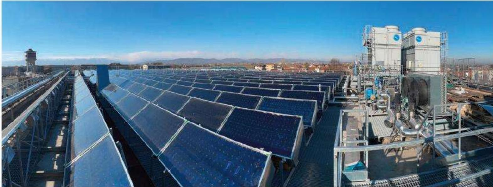
Solar process heat system for Martini & Rossi with a capacity of 0.42 MW<sub>th</sub> and equipped with high-vacuum flat plate collectors in Turin, Italy
