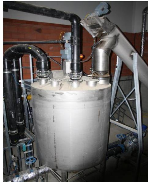
Figure 4: Système de "feedcontrol". Source: EnviTec
